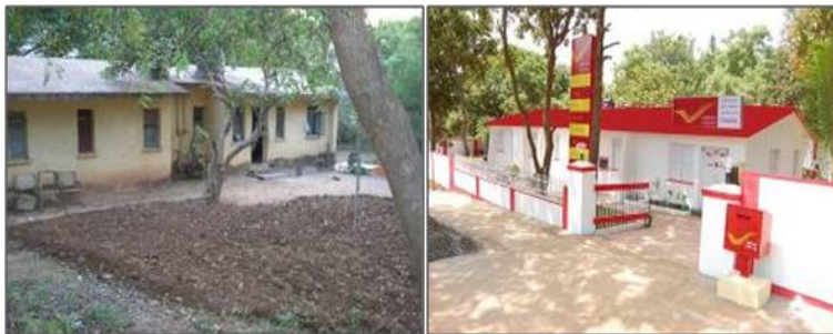
Before and After : Dwaraka Tirumala Post Office, Andhra Pradesh, India
